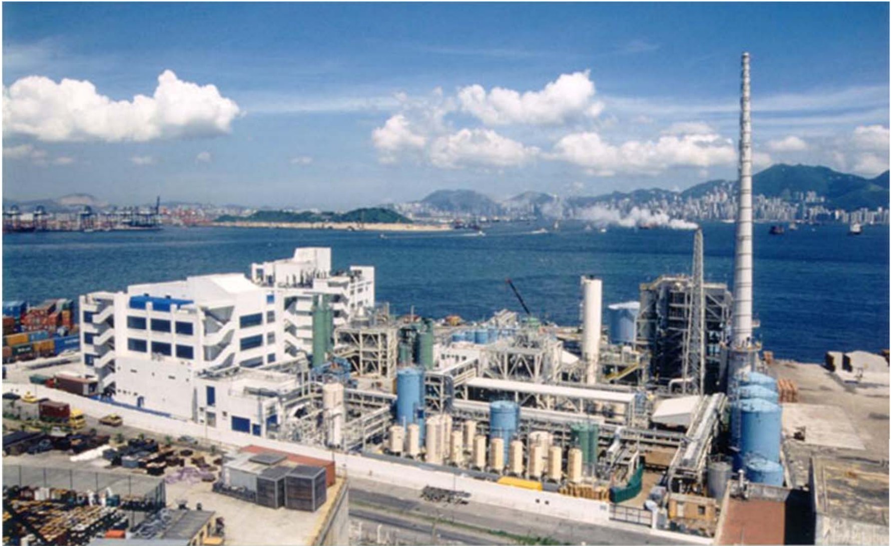
Hong Kong Chemical Waste Treatment Center - Where M-WTE was first conceptualized in the late 90's
