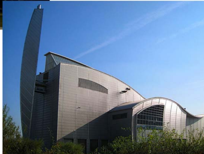
Sludge Incinerator East London UK
