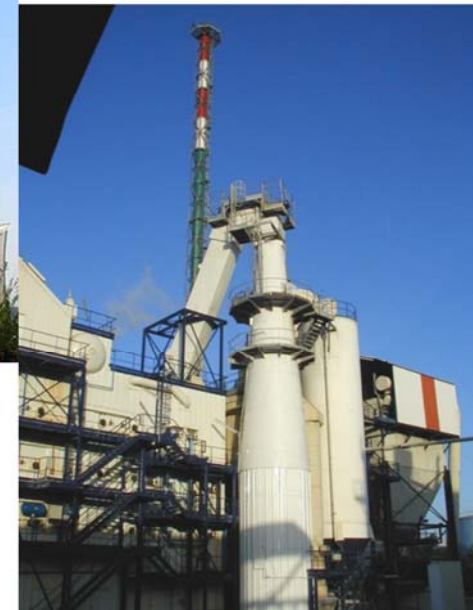
Hazardous Waste Incinerator Limay France
